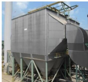
Gambar 2.1 *Electrostatic Precipitator*
