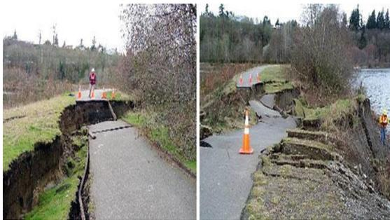
Gambar 4. *Lateral Spreading*
