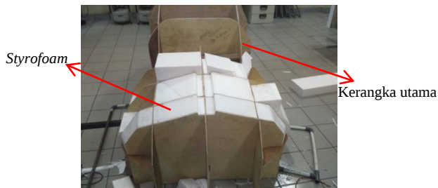
Gambar 9 Proses pengisian Styrofoam .
