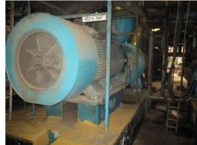
Gambar 2.1 IP 923-UE303-M1 *Primary Screen Pump*
